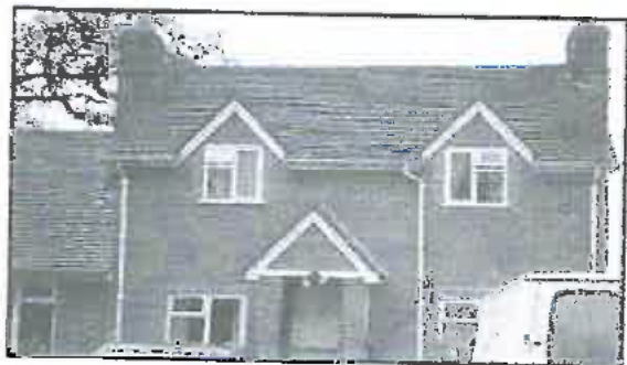
The Former Bowman's Cottage in Sandy Lane Pictured in Recent Years
